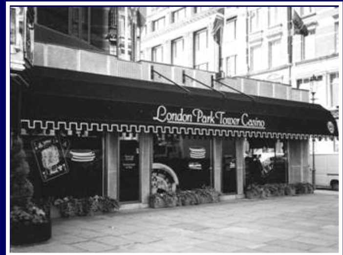
Park Tower Casino - 2000
